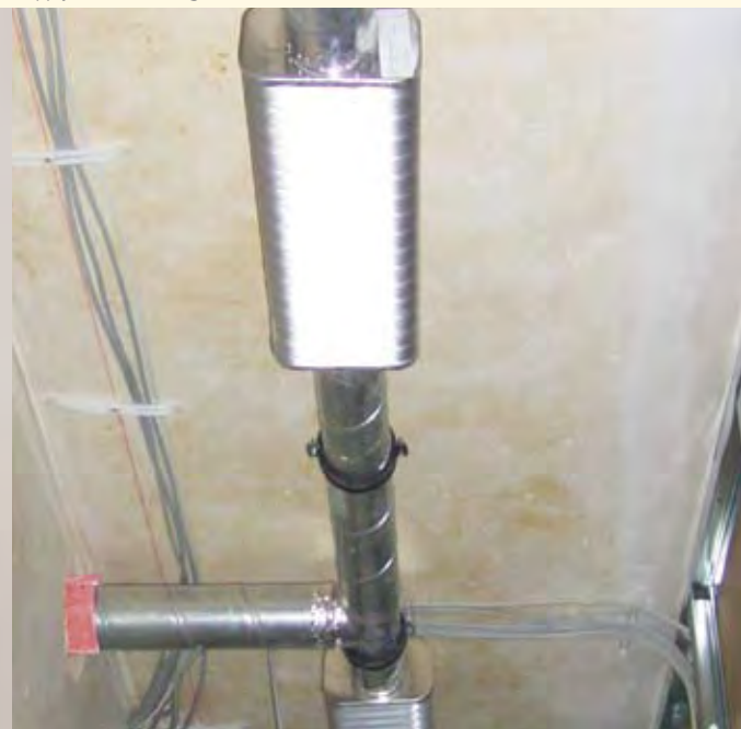
Supply air duct during construction
