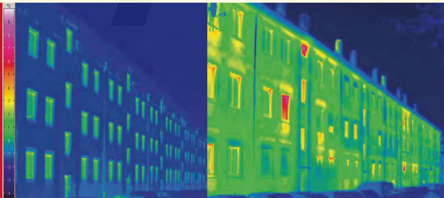
Thermographic image after (left) and before (right) refurbishment.
